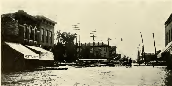
LOOKING SOUTH ON KANSAS AVENUE, SHOWING WRECKAGE ON NORRIS STREET
