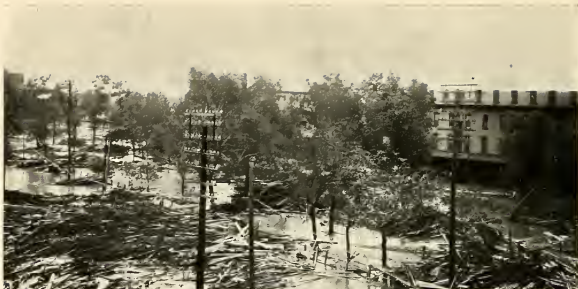
LOOKING SOUTHEAST FROM NORRIS STREET, SHOWING UNION PACIFIC DEPOT AND PARK
