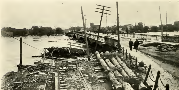
MELAN ARCH BRIDGE, AFTER WATER HAD FALLEN SIX FEET
