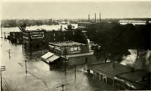
GENERAL VIEW OF THE FLOOD,—LOOKING NORTHEAST FROM PARKHURST-DAVIS BUILDING, SHOWING NORTH TOPEKA AND SANTA FE BRIDGE
