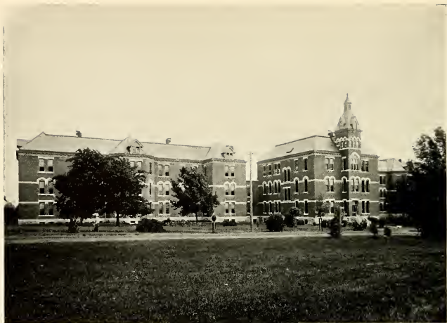
BUILDING FOR INCURABLES, STATE HOSPITAL FOR THE INSANE
